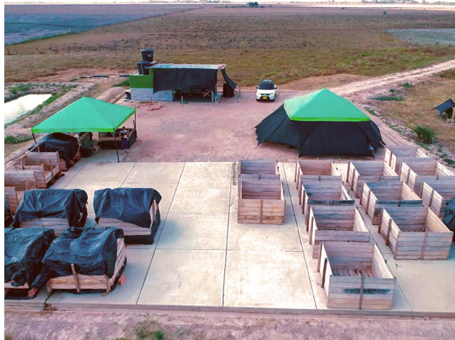
SACOOP composting centre
